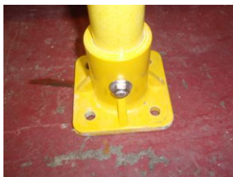
Figure 2: SMC post bases: (a) for a circular cross-section post
